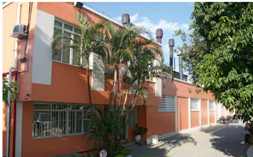
The new premises of Sprimag Brasil is significantly larger than the previous Building pictured here.
